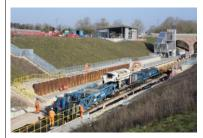
The new station being developed at Winslow is taking shape and is due to be completed later this year. Platform construction began a year ago, with more than 500 pre-cast concrete units being lifted into position within the new railway cutting before work could begin on the station building itself.
